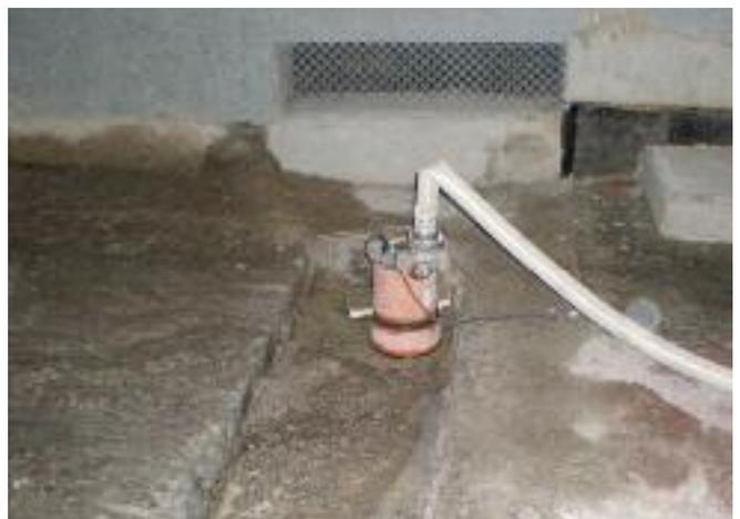
In the event of abrasive and corrosive utilization, stronger wear and tear will take place naturally in certain components. With regards to the above application wear and tear can take place mainly in impeller, agitator, suction plate, shaft sleeve, oil ring, mechanical seal, pump casing, strainer, motor casing and discharge coupling. Depending on the working conditions the lifetime of those parts might vary significantly and can be shorter than the legal warranty period.
