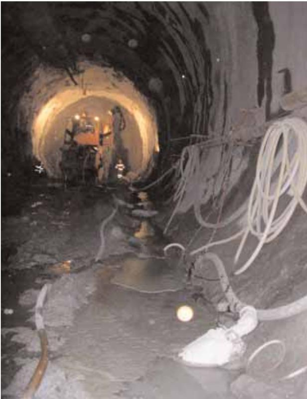
The "Sedrun Section" of the Gotthard Basistunnel encompasses two tunnels that are each 6,2 kilometres long and supplied through a 800m deep mine shaft. Two tunnels are at the base of the shaft and each breaks through to the north and south in the conventional manner. The project tunnels through the unstable rock of
