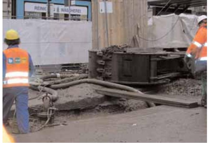
Slot wall with pressure lines
