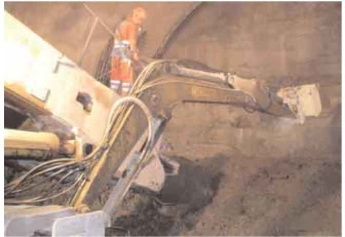
Portal with partial cut machine in operation
