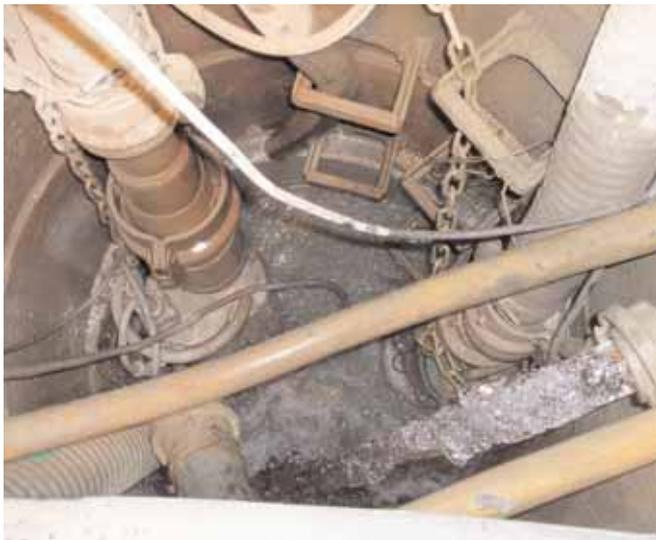
Collecting shaft with KTZ47.5 and KTZ35.5 in operation in snore mode
