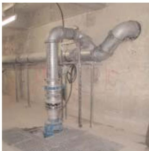
In the event of abrasive and corrosive utilization, stronger wear and tear will take place naturally in certain components. With regards to the above application wear and tear can take place mainly in impeller, suction plate, shaft sleeve, oil ring, mechanical seal, pump casing, strainer, motor casing and discharge coupling. Depending on the working conditions the lifetime of those parts might vary significantly and can be shorter than the legal warranty period.
