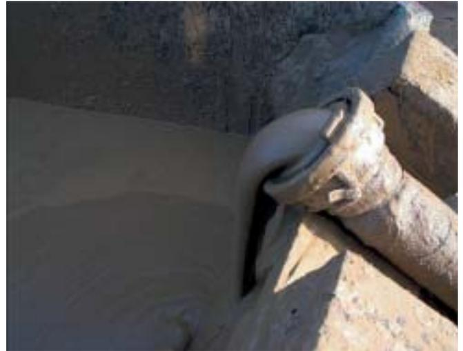
pump which could be used also during pressing. Transporting off was simple as it was possible to pump the drilling material directly into the containers provided. No tank truck was necessary.
